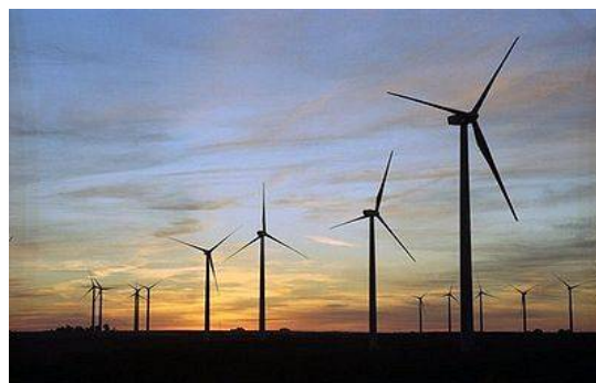
Wind Energy system
