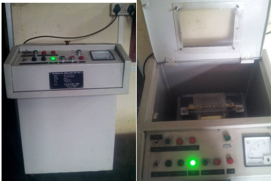
Fig: Transformer Oil Testing
