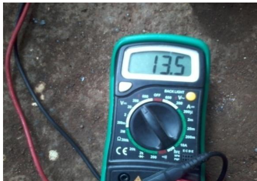
Generator output with load (Battery)
