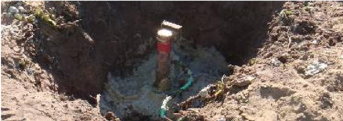
Fig 3. Bentonite Earthing
